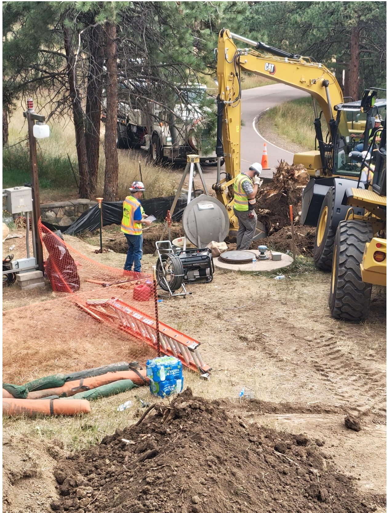
Potholing to gently remove soil around the pipe was also performed and the pipe was exposed late that evening. Troubleshooting began the following morning and the replacement check valves were installed by Direct Discharge.
