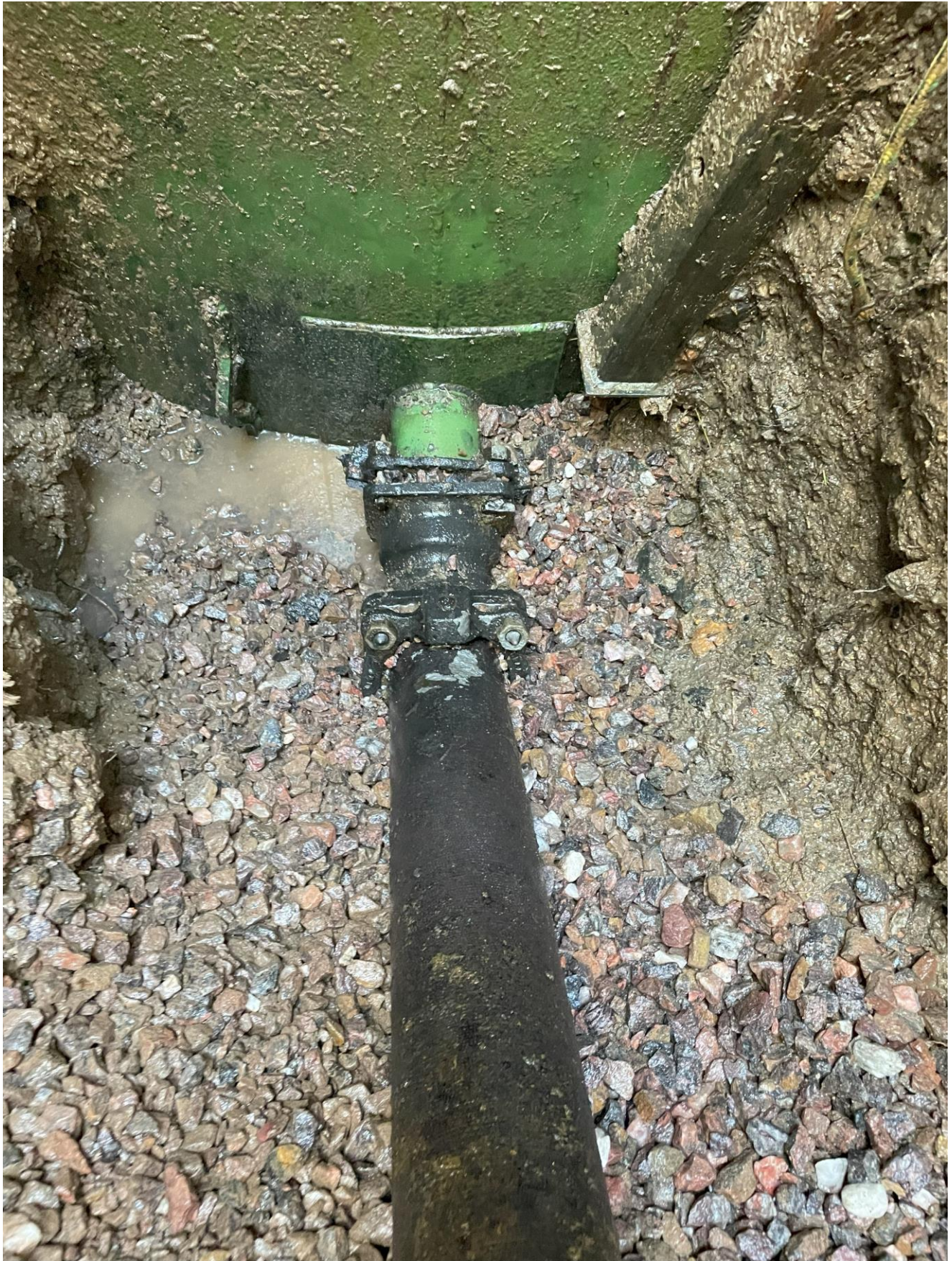
August 28 th the repairs were completed with proper bedding and new mega lugs joints, elbow joints, and sections of ductile iron pipe. Also, it was discovered that boulders were used as thrust blocks and were removed. Proper concrete poured thrust blocks were added.
